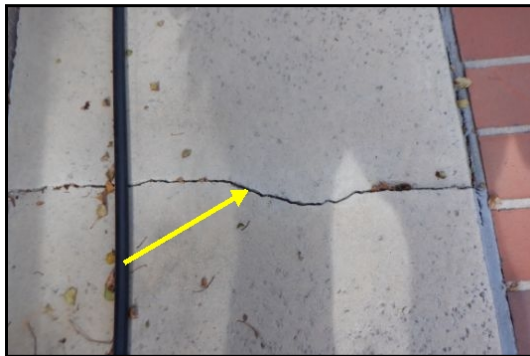
Moderate cracks
