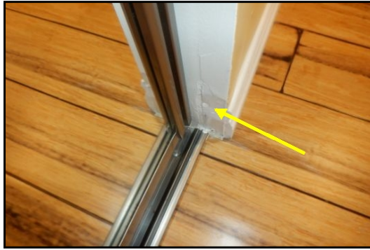
Peeling paint/deterioration
