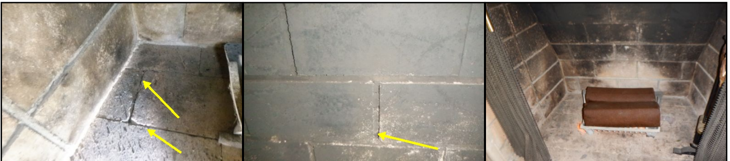
Deteriorated mortar
