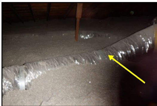
Duct work lying on ceiling joist
